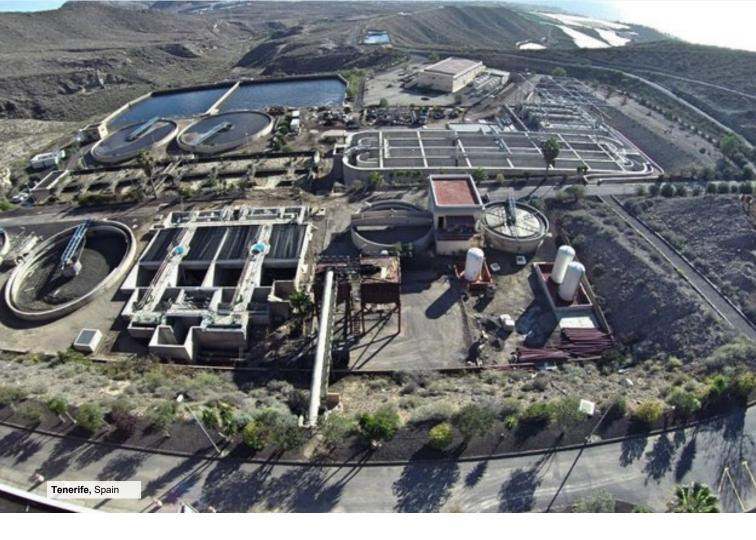
Arona-Este Sanitation **System**  Execution of the Arona-Este Sanitation System as well as the construction project of the collectors and impellers associated with the Montaña Reverón WWTP. A comprehensive sanitation and purification system for urban wastewater has been built, as well as regenerating the treated wastewater so that it can be reused for agricultural irrigation.
