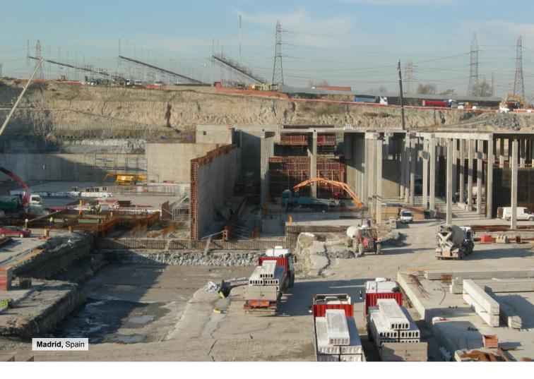
Construction of the "Butarque" storm pond The "Butarque" storm pond has 400,000 cubic meters of reservoir capacity, with a surface area of 40,000 square meters.
