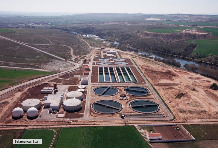
South general wastewater treatment Plant and Water filtration station The works include the construction of the south general wastewater treatment plant (WWTP) in Salamanca. The wastewater network was also extended to transport waste from the location of the old WWTP to the new plant.
